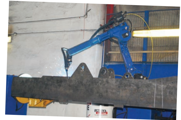
Above: Robot Welder
